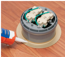
Wire receptacles. Seal underside of flange with silicone sealant if desired (not included).
