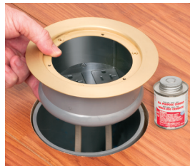
After installing flooring secure leveling ring assembly to floor with PVC cement applied around flange.
